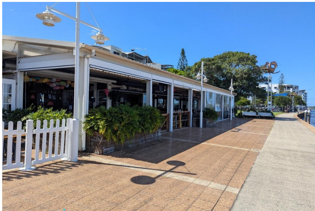
Figure 2: Paved area adjacent to southern side of The Wharf Bar and Restaurant
