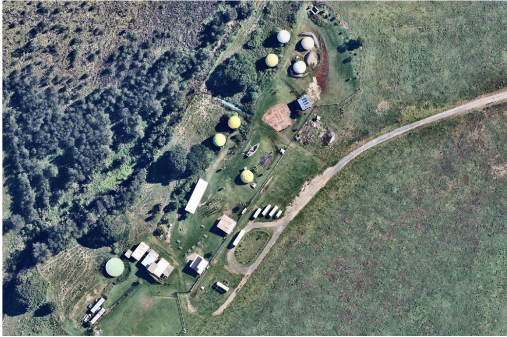
Figure 3: Aerial Imagery Showing School Structures
